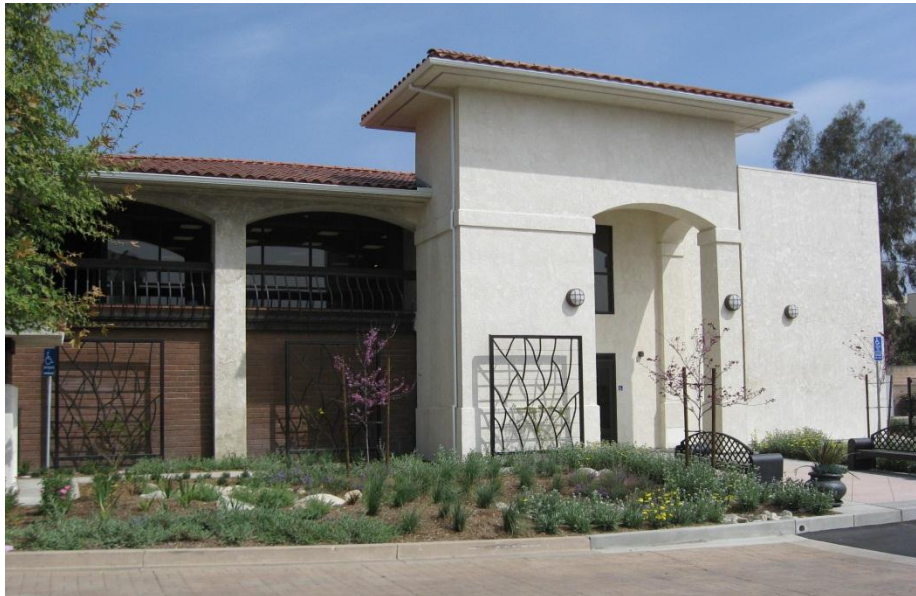
A view of the Monte Vista Water District main office building's new exterior.
